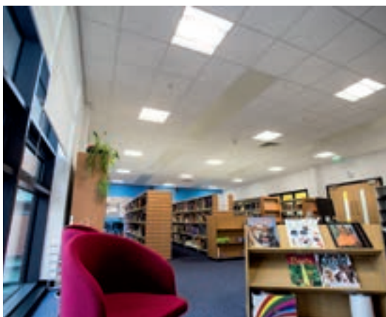
THERMATILE PLUS Radiant Ceiling Panels at Crown Hills School, Leicester
