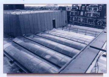
Continuous Barrel Lights manufactured from GMS or aluminium are available to suit any roof opening. All vent options, insulation and burglar bars are available. Top components are manufactured in Single or Double Skin and are available in Clear, Opal or Bronze PVC; High impact resistance Clear, Opal or Bronze Polycarbonate.
